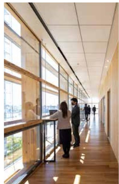
Inside, CLT-paneled walls and narrow outer wood members create a workspace with the warmth of wood and a sense of openness.
