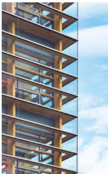
The double skin facade supported with laminated wood has a low environmental impact and gives the impression of wood from the outside.
